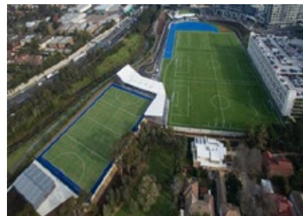
Photo 4: Football, AFL and Cricket - St Kevin's College Vic (installed by Tuff Turf)
