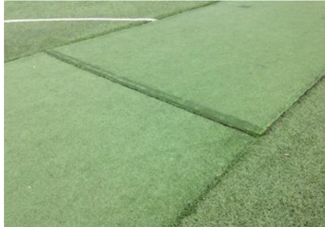
Photo 27: Maintenance between two different surfaces means that two different schedules or plans to ensure success are required
