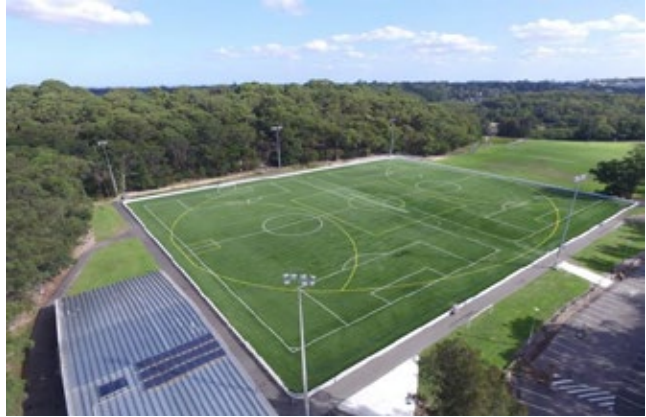
Photo 29: Blackman park, Lane Cove NSW - Installed by Team Sports (Source - Lane Cove Council)
